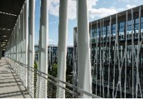
UHPC ribbed vaulted
